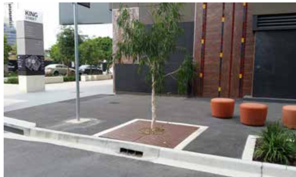
Use a tree grate to avoid the fall hazard. Location – King Street, Bowen Hills
