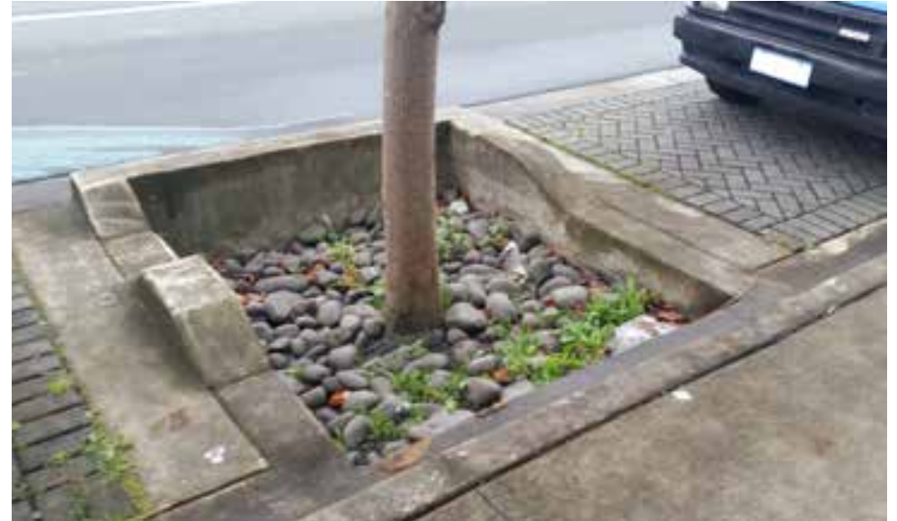
Rocks are known to capture sediment and propagate weeds. Location- Warnboet Ln, Auckland
