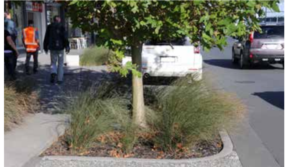
Use flush kerbing to divert sheetflow into street tree pit. Location - Ansett Place, Auckland
