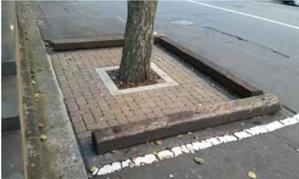
Concrete collar can restrict tree growth. Timber sleepers can age poorly. Location - Market Place, Auckland
