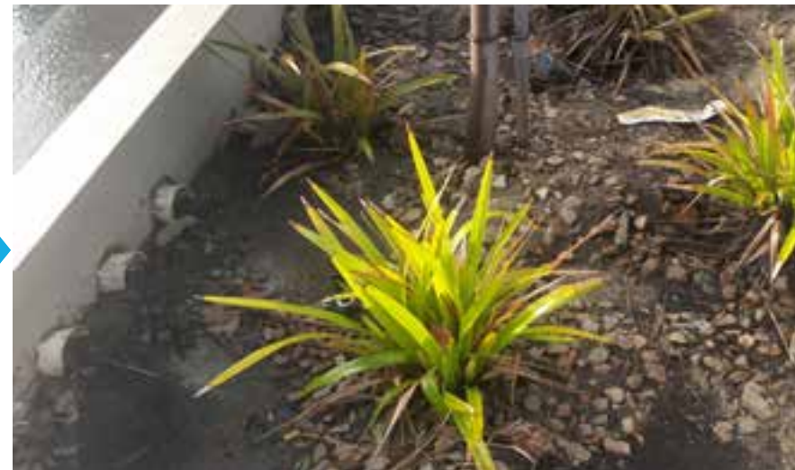
Problem: Inlets become blocked with sediment and leaf litter
